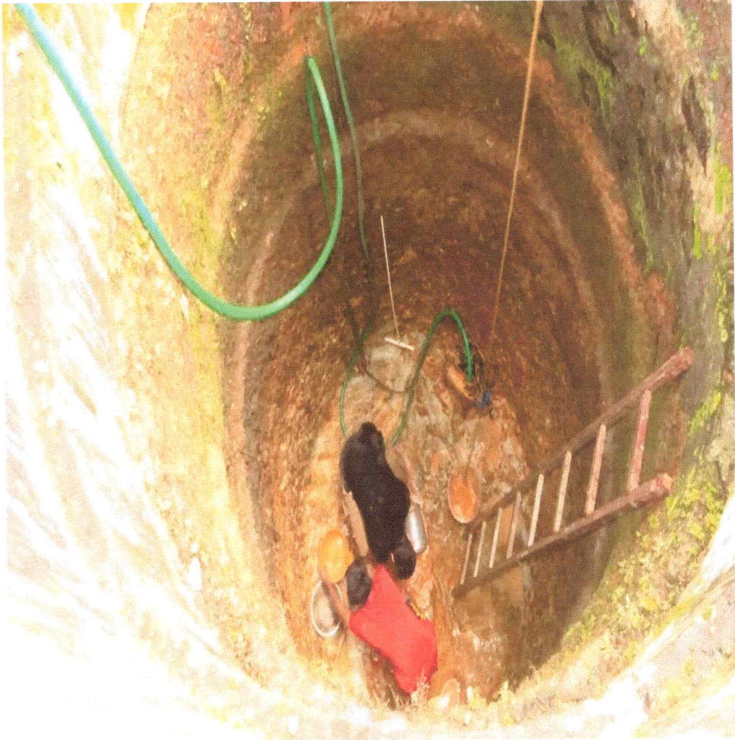
Well Cleaning Program
